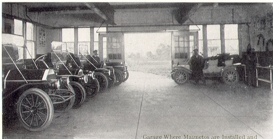
Garage Where Magnetos are Installed and Employes' Cars are Kept
